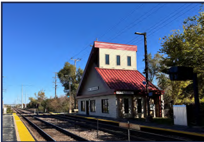
FIGURE 25: NORTH CHICAGO METRA STOP
