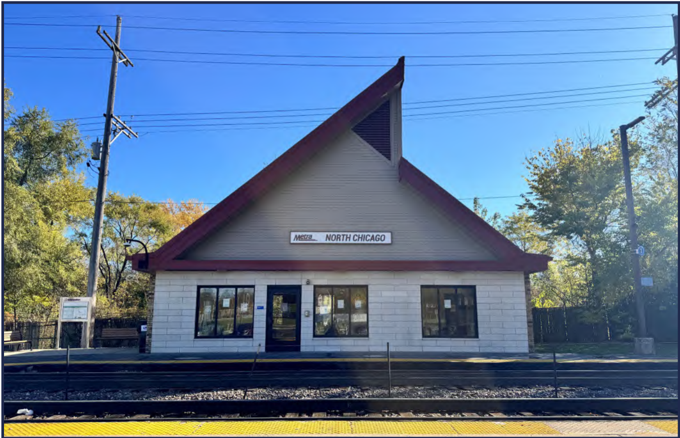
FIGURE 14: NORTH CHICAGO METRA STOP
