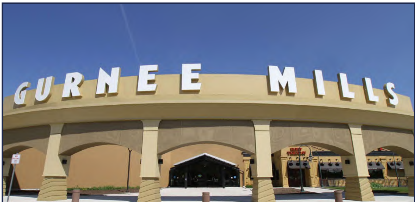
FIGURE 17: GRUNEE MILLS SIGNAGE
